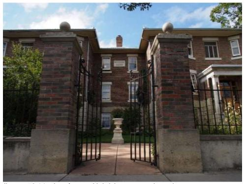
(Image #2.14 – Iron fence with brick support columns)
