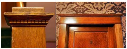
(Image #3.3 – Typical oak detailing on newel post and door casing)
